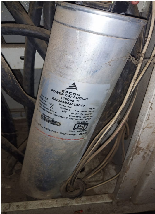
Image of capacitor at new building panel board
